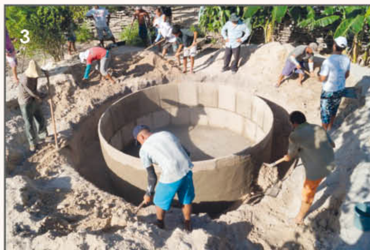
Aterrando as placas do fundo (1,5m).
